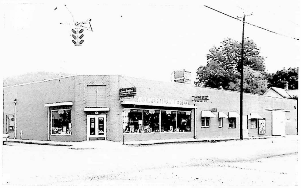
MAIN STORE BUILDING
